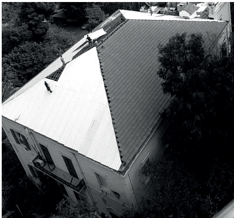
Figure 3. Following the explosion at the port in Beirut on 4 August 2020, the Blue Shield worked with partners in Lebanon to secure more than 30 cultural buildings (libraries, museums, archives etc.) and to stabilise two major historic buildings. © Biladi.
